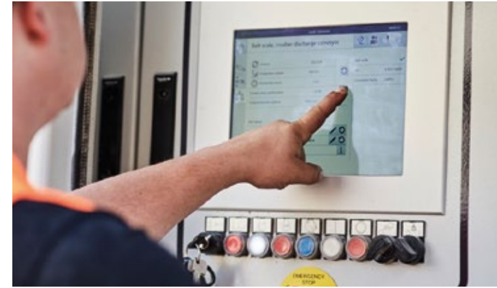
> Trigger the "Lock rotor" command via SPECTIVE
